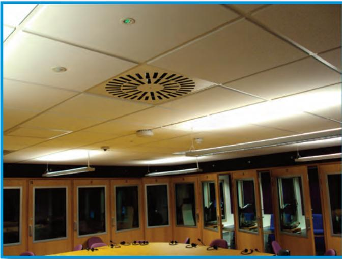
Eaton-Williams® COLMAN® range of ceiling grilles were also extensively used. The 'D' Series of fixed circular swirl diffusers which offer a high level of induction due to the angle of the blades and provide warm or cooled air to the required space are used for extracting air in the language labs. The 'G' Series of return air grilles were selected for both wall and ceiling applications.
